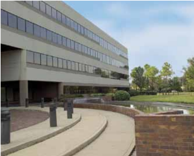
HCC Alief Campus 2811 Hayes Road Houston, TX 77082
